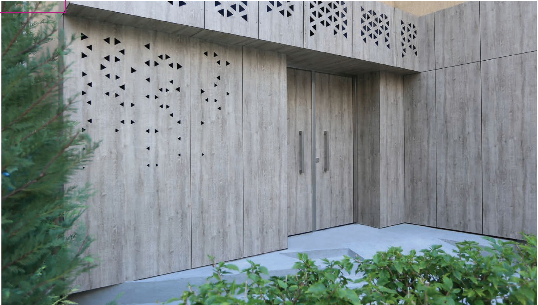
EXTERIOR WALL CLADDING AND SECURITY DOOR
