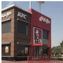
01 EXTERIOR WALL CLADDING
